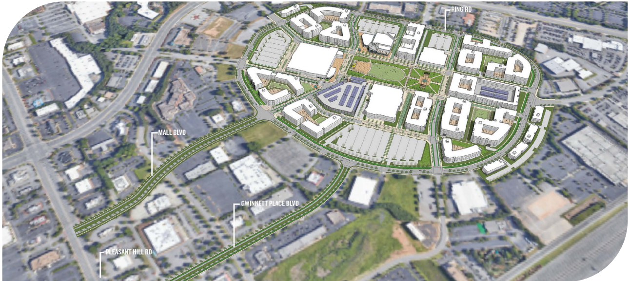
At the former Gwinnett Place Mall site, a reimagined mobility hub concept and strategy bring new life to an old shopping mall site through enhanced and appropriately scaled TOD.
